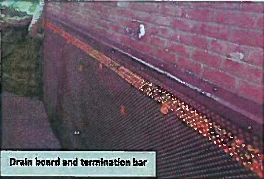
Black elastomeric membrane is applied
