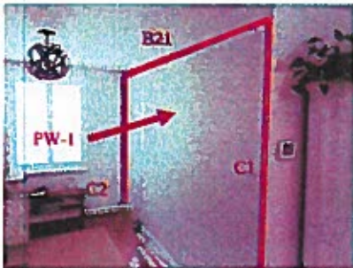
Picture 5: Partition wall to be removed PW-1 around kitchen (view from dining)
