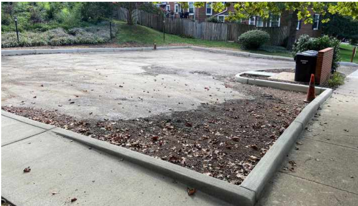
The above photo taken at parking lot 34 (4828-4836 S. 29 th Street) demonstrates how minor adjustments can be made to improve traffic flow and in this case, add an additional parking space by extending the curbs out slightly from their original location.
