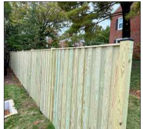
PHOTO BY MARK JOHNSON Phase I of the perimeter fence.
