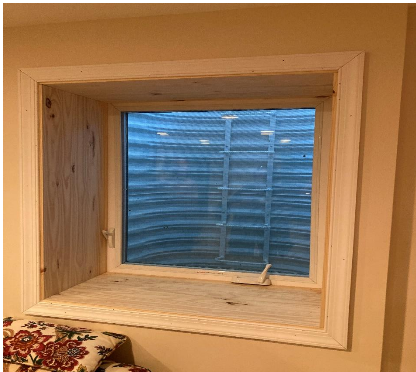
Figure 2 Egress window inside view
