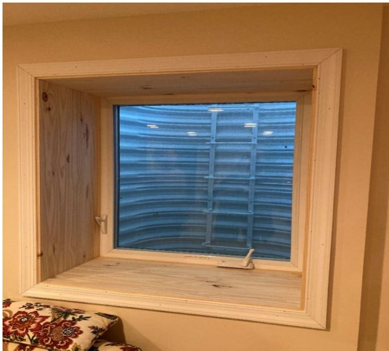
Figure 2 Egress window inside view
