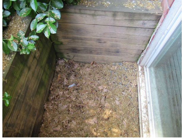
Photograph #6: Timber window well at previously approved location
