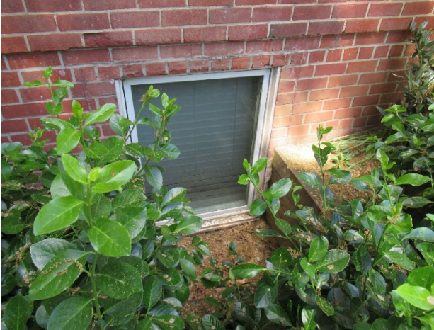
Photograph #5: Egress window at previously approved location
