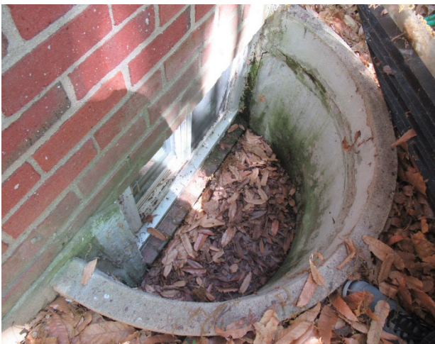
Photograph #3: Concrete window well
