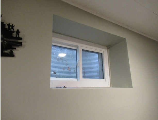
Photograph #1: Typical interior window opening
