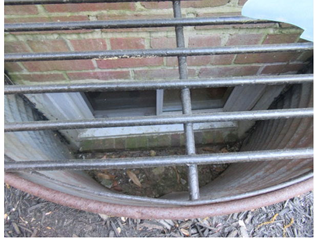
Photograph #2: Window well with galvanized steel and steel bars over top
